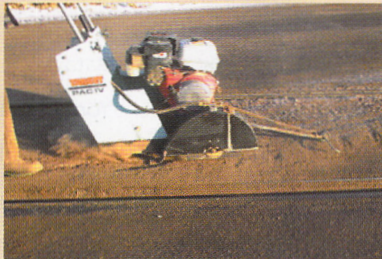
Diamond saws enable fast, focused street repair without noisy and destructive jackhammers.
