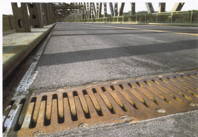
Expansion joints on a bridge allow the steel supports to expand in hot weather without buckling.
